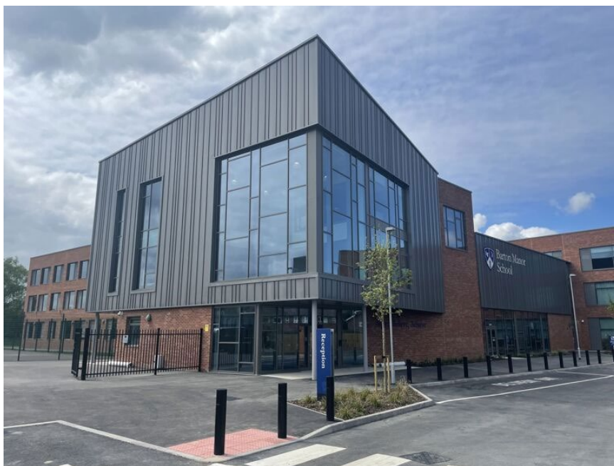
Entrance block to new school
