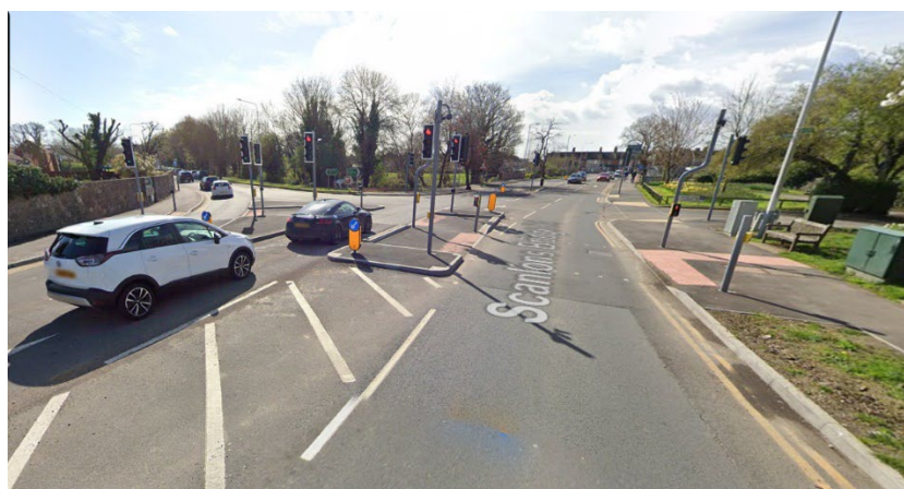
Junction layout after works
