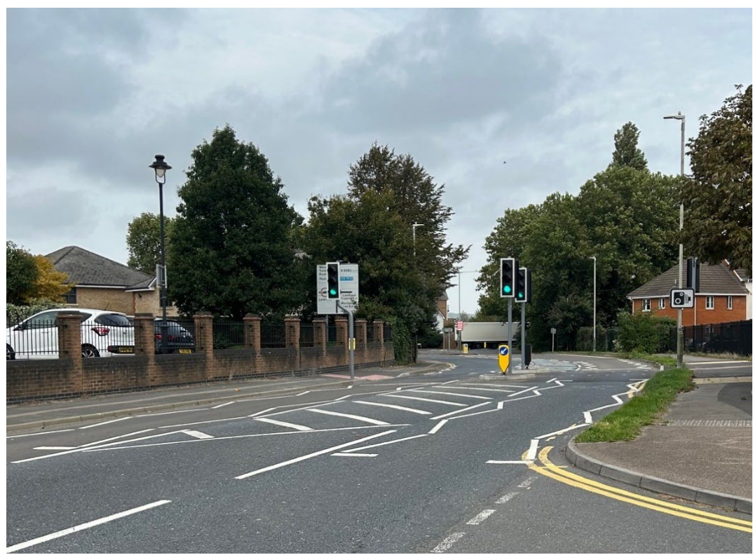
New signalised crossing
