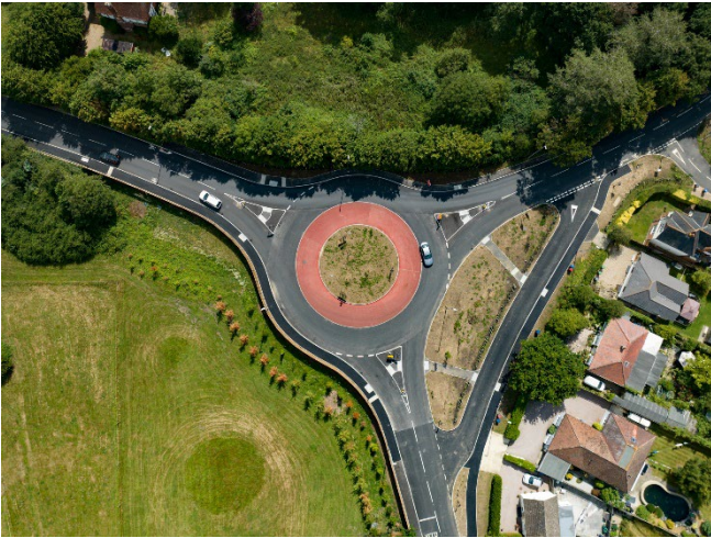
Aerial view of new roundabout 1
